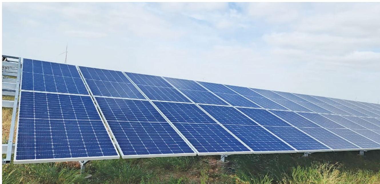
Use of bifacial solar modules at Clean Solar Power (Bhainsada) Private Limited
