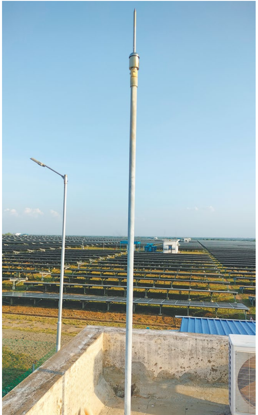
Lightning Arrestor at WREL's project in Trichy district, Tamil Nadu
