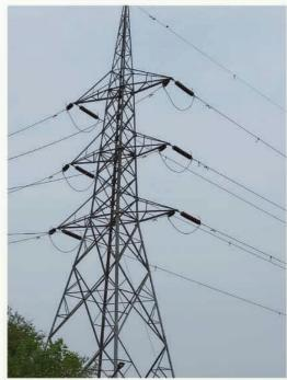
Bird diverters installed on powerlines falling in GIB sensitive habitats
